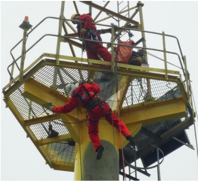
Spray coating steelwork after blasting completed.
