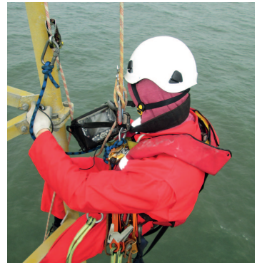
Once all work was completed, NDT inspections on the Mast were carried out during another visit. This included the tightening of all bolts on the structure.
