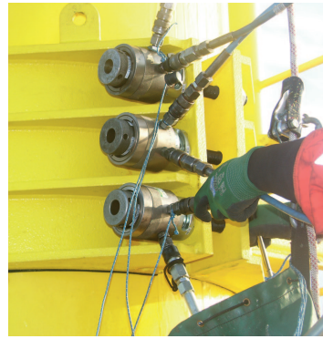
Trained Abfad personnel tightening clamps using Hydratight hydraulic equipment.
