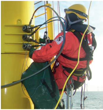
Trained Abfad personnel tightening clamps using Hydratight hydraulic equipment.
