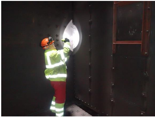
Site Staff member performing inspection task
