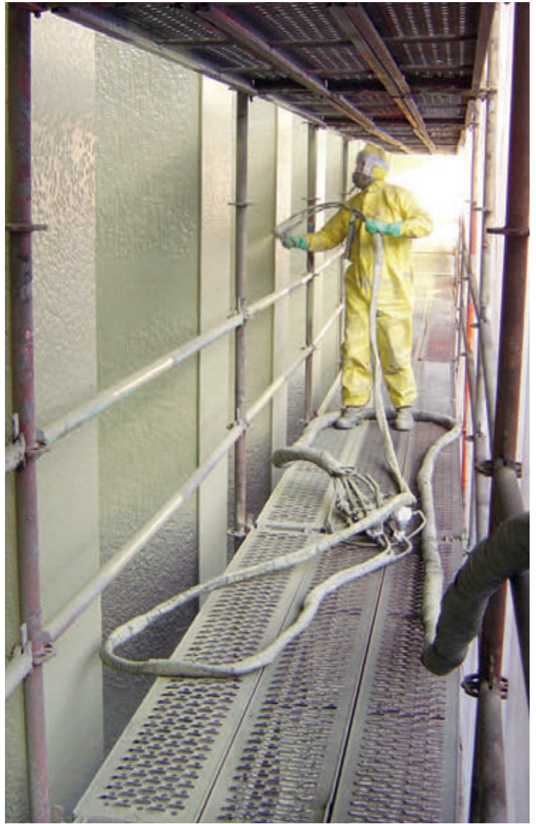
Fast set Urethane applied to cargo hold bulkheads and ladder sections to a thickness of 3mm (3,000 microns) in 1 single application.
