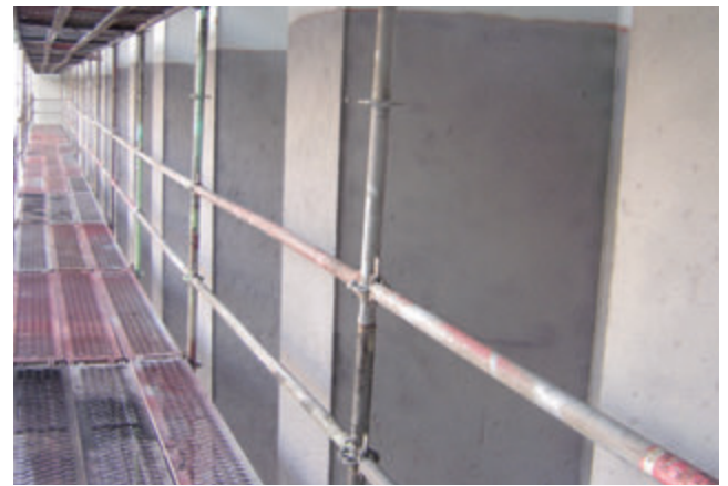
Corrugated bulkheads blasted to SA 2.5 standard prior to coating application.
