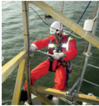
Once all work was completed, NDT inspections on the Mast were carried out during another visit. This included the tightening of all bolts on the structure.
