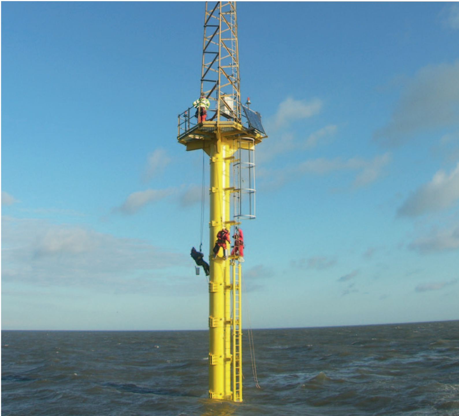
Abfad personnel performing finishing touches and final checks on Met Mast at Scroby Sands, Great Yarmouth.
