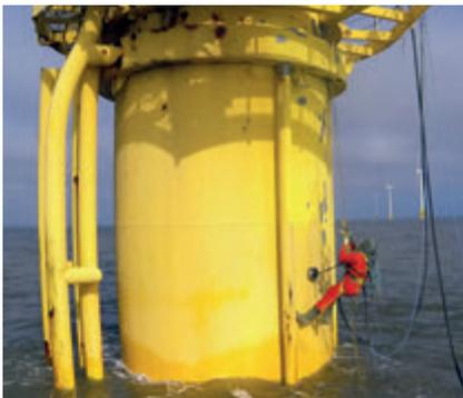
Blasting structure by means of rope access with unique magnet system
