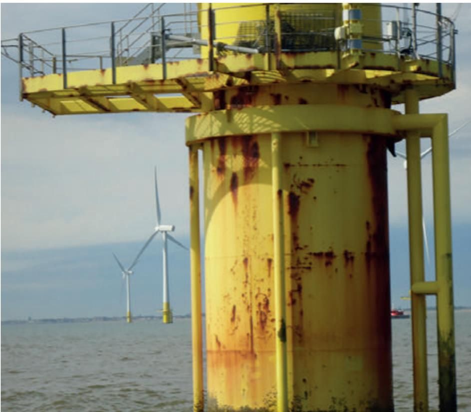
Existing condition of Monopile steel, detailing corrosion to structural beams below gratings and main body of structure
