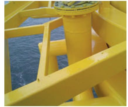
Close up of new protective coating, applied by airless spray unit, applied to required thickness to main structural steel below gratings
