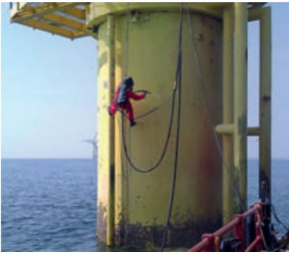
Rope access blasting to SA2.5 standard with sound paint profiled to take new spray coating
