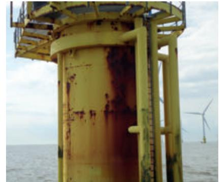
Picture detailing severe corrosion to main steel sections below gratings
