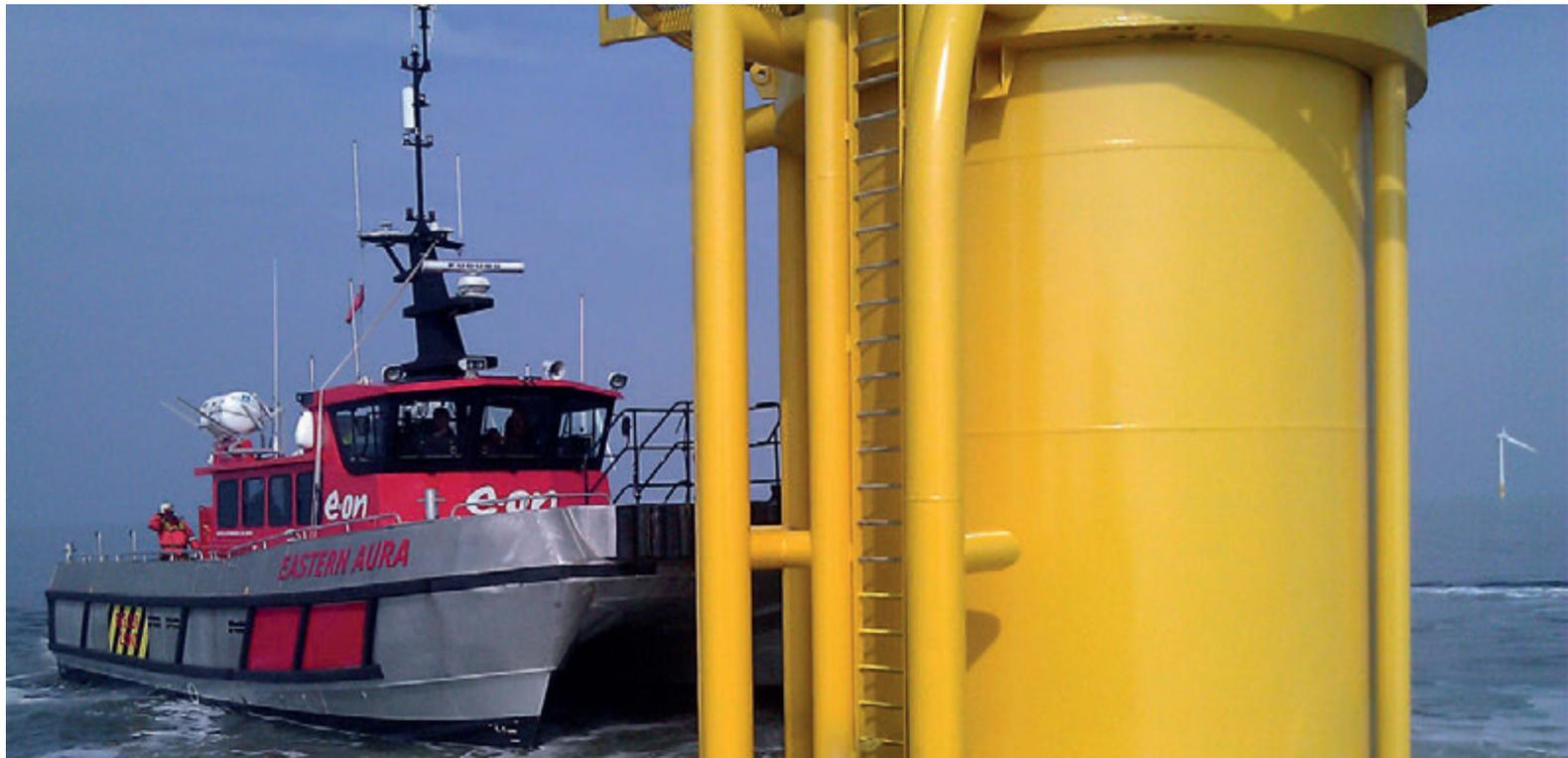
Picture detailing completed Monopile structure which has been fully blasted and protected by nominated coating from walkway grating beams to sea level, including all pipework
