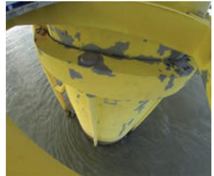
Work in progress on Monopile with sections of corrosion removed and existing coating profiled and feathered back in preparation for spray coating
