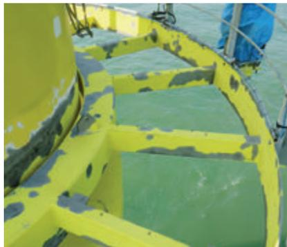
Picture detailing all corrosion removed to blast standard SA2.5 with sound paint profiled to take new spray coating
